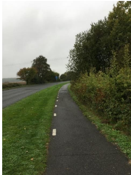
Photograph 5: Existing Footway / Cycleway on Peak Lane
